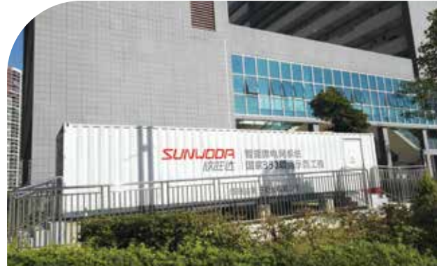
National "863 Subject" 250kW/580kWh Campus Smart Microgrid Key Technology Research and Integration Demonstration Project
